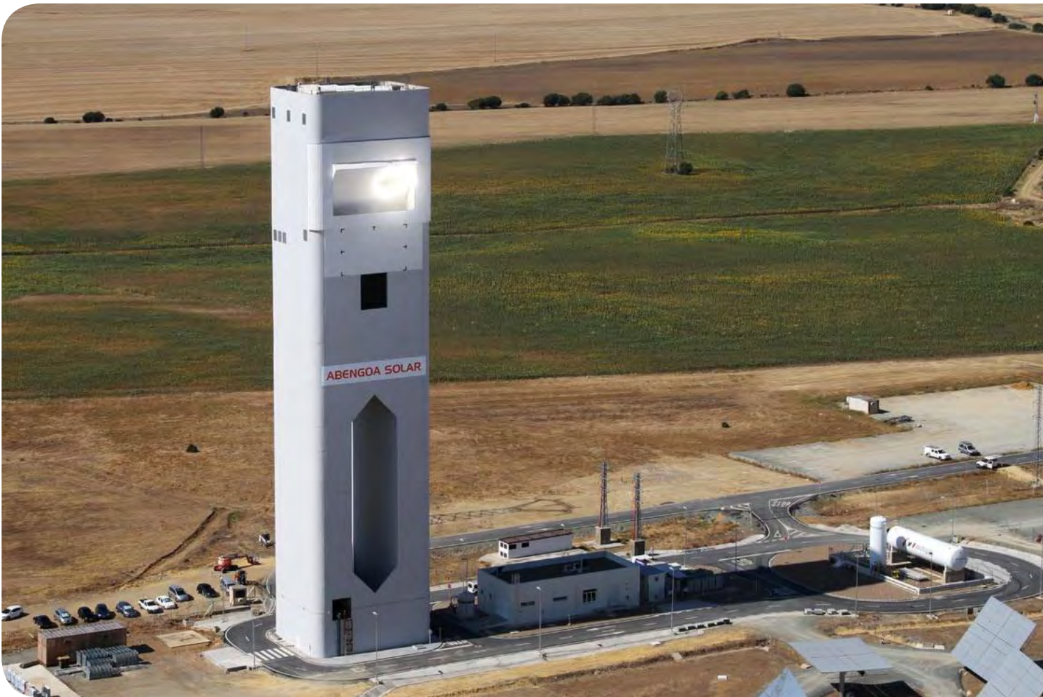
Solugás pilot plant, Seville, (Spain).
